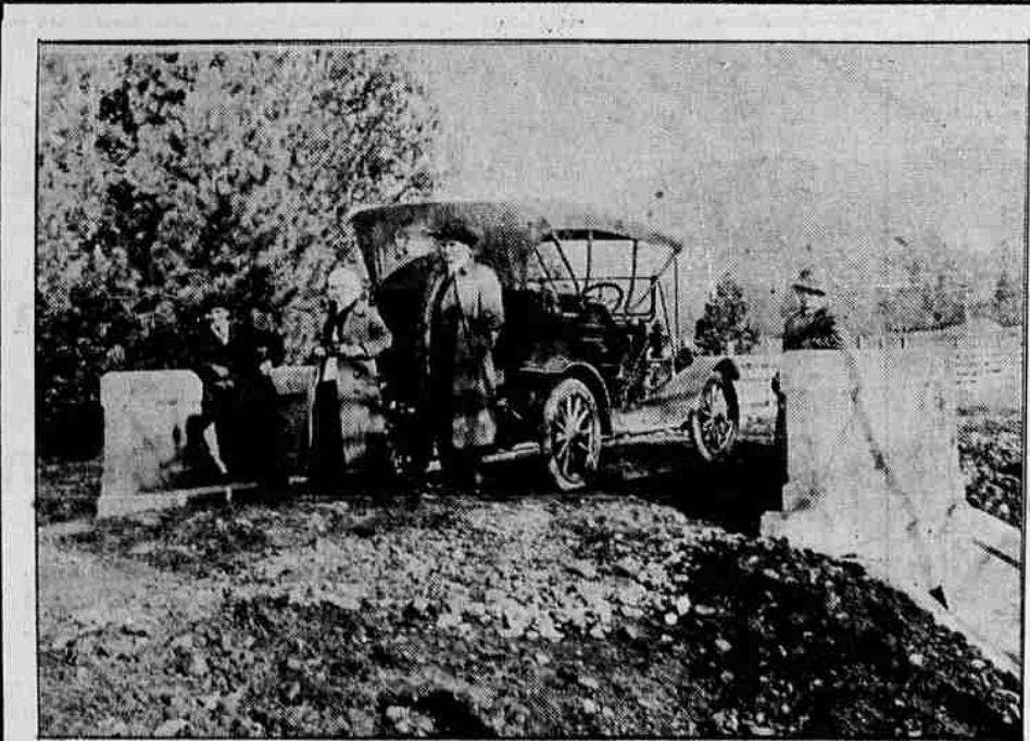
CULVERT, ON POSTAL HIGHWAY
