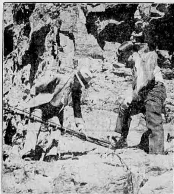
Maj. F. J. Pomeroy of the Arizona national guard and Herbert H. Hotchkiss, secretary to Gov. E. B. Moerz, inspect a cable claimed to have been anchored on the Arizona side of the Colorado river by the Metropolitan Water District of California preliminary to the construction of the Parker diversion dam. Governor Moerz opposes the project and has said he will call out the national guard to prevent its construction. (Associated Press Photo)
