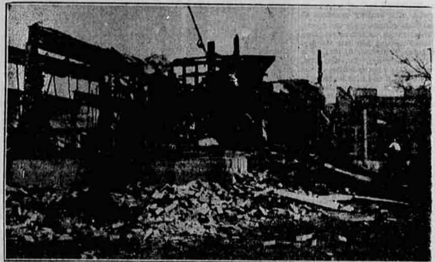
A midnight fire that razed the three-story Longview, Tex., hotel resulted in the deaths of three persons and injuries to many others as they jumped from the blazing structure. Photo shows ruins a few hours later. (Associated Press Photo)
