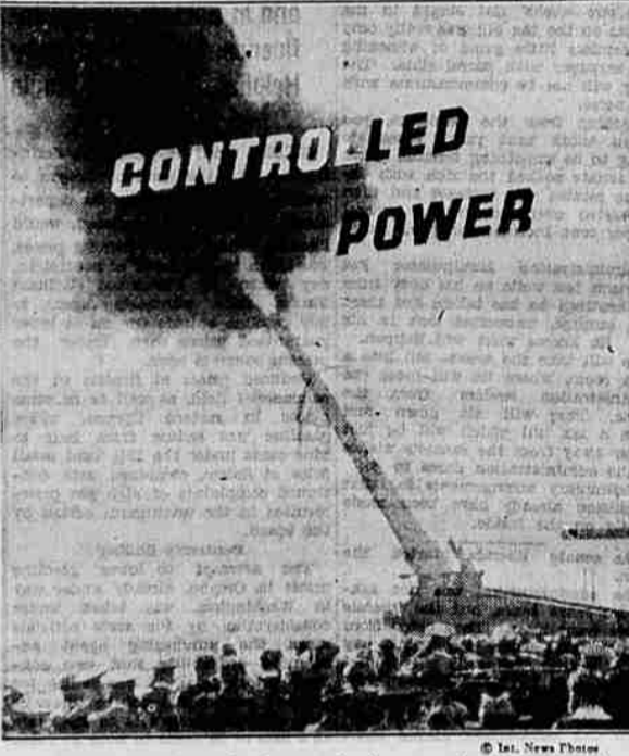
Firing the new model 16-inch gun at the Army proving grounds. This gun is mounted on a Barbette carriage and is loaded and directed by electric power. The shells used weigh 2,100 pounds and the gun has a range of 34 miles because the power of the slow-burning smokeless powder used is controlled. Gilmore Oil Company engineers say this same Controlled Power principle is now applied to gasoline. Power is concentrated and sustained on the piston head for the full length of the stroke. (adv.)
