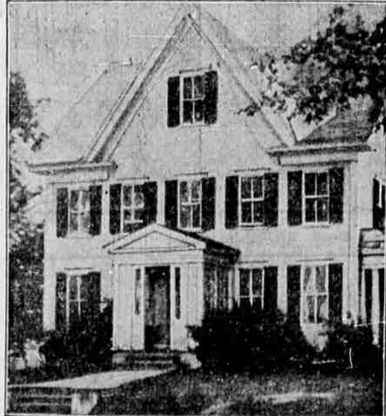
Nine Dartmouth college students died in the Theta Chi fraternity house (above) at Hanover, N. J., from carbon monoxide gas which swept through the 16-room house after a coal gas explosion apparently blew open the furnace doors and disconnected a chimney pipe. (Associated Press Photo)
