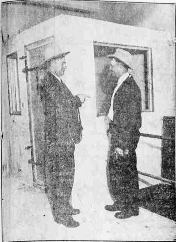
Warden A. G. Walker (left) of the Arizona state prison in Florence is pointing out the observation window of the nearly completed lethal gas chamber which will be used for executions in the future to Yard Captain Bert Polly. Arizona is the third state to adopt this method of putting condemned persons to death. The chamber is in a small room above the condemned cell block and was formerly used for handbills. (Associated Press Photo)
