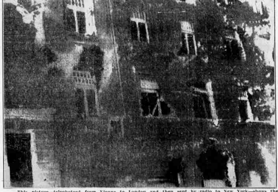
This picture—telephotoed from Vienna to London and then sent by radio to New York—shows the damage done to the Karl Marx apartments in Vienna when government howitzers shelled the socialist stronghold, killing and injuring many. The holes torn in the front of the building by the shells may be seen. The Karl Marx apartments, largest in Europe, were the scene of the bitterest fighting in the revolt. (Associated Press Photo).
