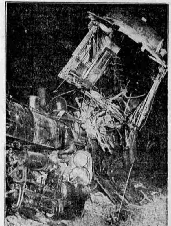
This was the dizzy sight which resulted after a passenger train collided with three switch engines, running tandem, near Fenton, Mich. No one was killed in the smashup, and only two trainmen were seriously injured. The passenger coach which bore most of the damage was uncoupled. (Associated Press Photo)
