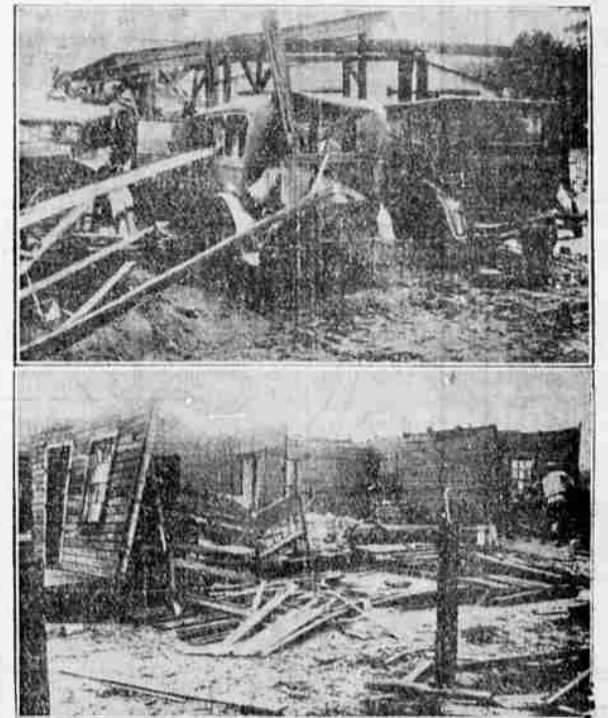
Here are two views of samples of the $100,000 property damage done by a storm which swept over Pensacola, Fla. At top are auto workers at a drydock, battered by flying planks. Below, ruins of a home in the residential section. (Associated Press Photos)
