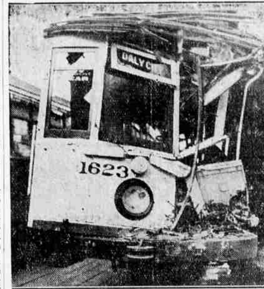
One of the two San Francisco street cars which collided at an intersection, injuring 34 persons, two perhaps fatally. A defective switch was blamed for the head-on crash. (Associated Press Photo)
