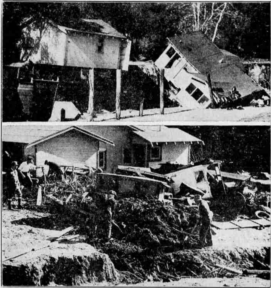
Here are two Los Angeles scenes taken as the army of workmen began its task of rehabilitating the flood-stricken area. The top picture shows a Verdugo Woodlands home in which a family of five narrowly escaped death, as it appeared after the waters had subsided, leaving the structure toppled into a ravine. Below: Workmen removing the wreckage of 14 automobiles which were washed against the house during the flood.—(Associated Press Photos.)
