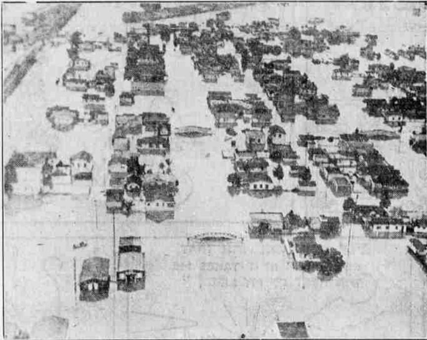
A striking air view of the half-submerged residential district of Venice, Cal., after flood water from torrential rains poured over the lowlands in which the town is located. Property damage in Southern California was estimated in the millions while 60 or more persons were killed. (Associated Press Photo)
