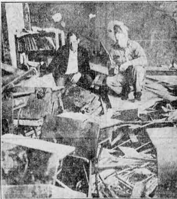
An 11-year-old boy and two negro janitors were fatally injured when the explosion of a basement boiler wrecked the fifth grade room of the consolidated school in Big Forest, Miss. Several other pupils were severely hurt. (Associated Press Photo)
