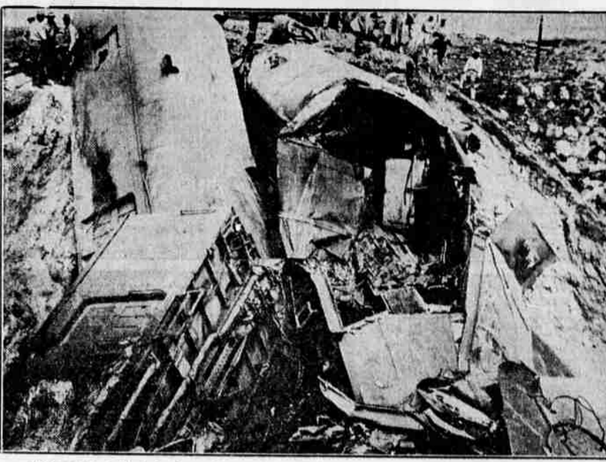
Plunging into a flooded arroyo when a section of the trestle washed out near Tucuman, N. M., the Golden State limited piled up as shown above. Eight persons were killed and two score hurt. (Associated Press Photo)
