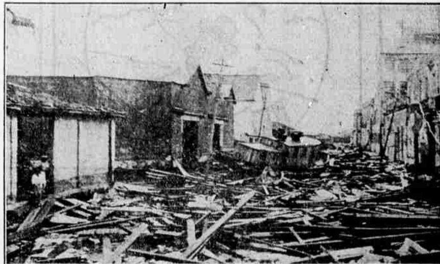
This picture shows a sample of hurricane damage in Cardenas, old Cuban town, where 30 were killed more than 100 hurt and hundreds of homes razed by the fierce storm which struck the western half of Cuba. Note the boat which was tossed into a debris-filled street. (Associated Press Photo)
