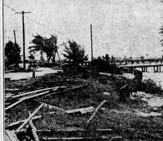
North Second street of Fort Pierce, Fla., is pictured strewn with wreckage tossed over it by waves during a tropical storm which whipped across the peninsula causing damage estimated at more than $1,000,000. (Associated Press Photo)
