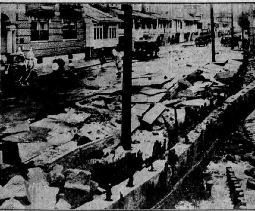
Striking with hurricane force the worst storm in years pounded the eastern seaboard killing at least a dozen people on land and sea and inflicting property damage running into many millions of dollars. Above picture taken at Atlantic City, N. J., shows a street near the beach battered to pieces by mountainous seas.
