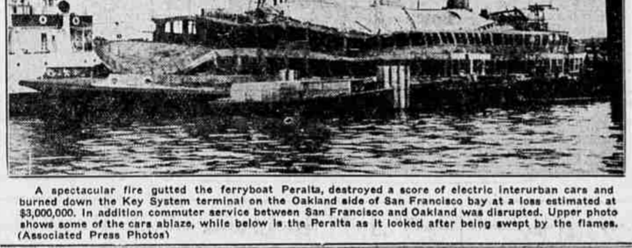
A spectacular fire gutted the ferryboat Peralta, destroyed a score of electric interurban cars and burned down the Key System terminal on the Oakland side of San Francisco bay at a loss estimated at $3,000,000. In addition, commuter service between San Francisco and Oakland was disrupted. Upper photo shows some of the cars ablaze, while below is the Peralta as it looked after being swept by the flames. (Associated Press Photos)
