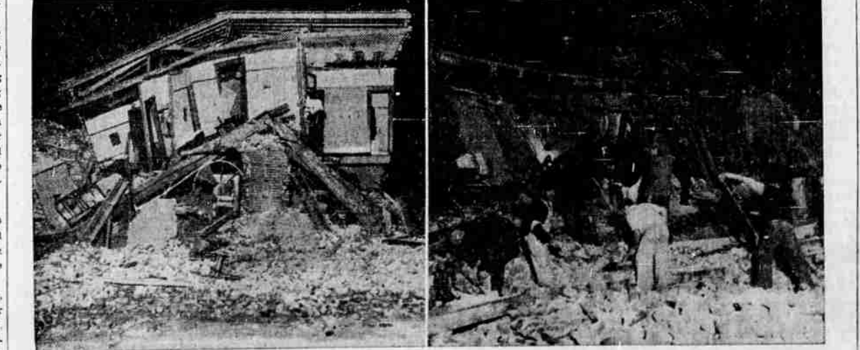
Two pictures taken at the scene show (left) a demolished hotel in Compton, Cal., from which seven persons escaped as it was torn apart by earthquakes. Right: Searchers working desperately in recovering the dead from the stockwell building in Compton, shaken down by a series of earthquakes which rocked Southern California. (Associated Press Photos)
