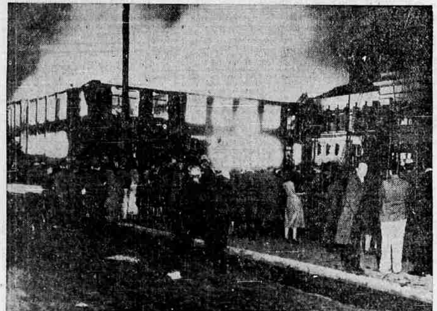
Associated Press telephoto rushed to this newspaper shows the Huntington Park, Calif., high school in flames after a large section of Southern California was rocked by severe earthquakes. A few hours after the tragedy 89 were reported dead with more than 2300 injured. The tremors were felt over an area 30 miles wide and 200 miles long.
