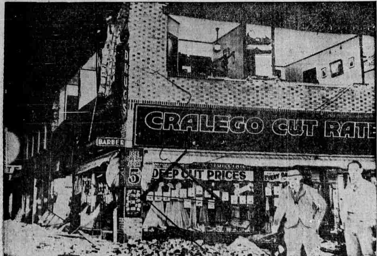
One of the buildings wrecked during a series of earthquakes in Los Angeles and vicinity. This wreckage of a Los Angeles store was pictured at Florence and Compton avenues shortly after the first shock, telephoned to San Francisco and rushed to this newspaper by the Associated Press.
