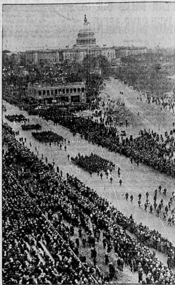
This striking air view of the Roosevelt Inaugural ceremonies shows the parade swinging from Constitution Avenue into Pennsylvania Avenue for the march to the White House. (Associated Press photo).
