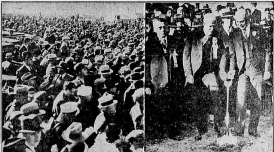
Just a small corner of the crowd that filled Crissy Field in San Francisco as ground was officially broken for the construction of the Golden Gate bridge on which actual work began several weeks ago. A gold shovel was used to turn the sod near Fort Mason. San Francisco's mayor, Angelo Rossi (right), and William P. Filmer, president of the bridge district, are shown turning the first earth while Chief Engineer J. B. Strauss (at Filmer's right) looks on. Because of the crowds the planned program was cut short. (Associated Press Photos)
