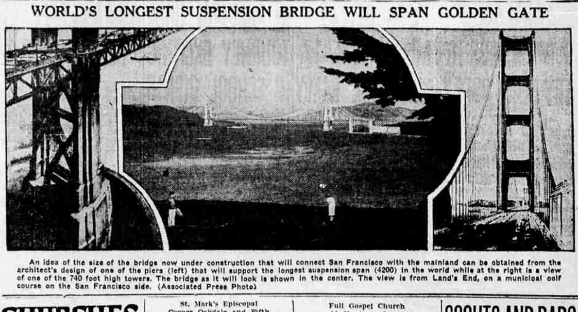
WORLD'S LONGEST SUSPENSION BRIDGE WILL SPAN GOLDEN GATE. An idea of the size of the bridge now under construction that will connect San Francisco with the mainland can be obtained from the architect's design of one of the piers (left) that will support the longest suspension span (4200) in the world while at the right is a view of one of the 740 foot high towers. The bridge as it will look is shown in the center. The view is from Land's End, on a municipal golf course on the San Francisco side. (Associated Press Photo)
