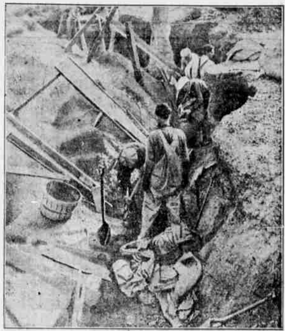
It was a case of every man for himself when coke was discovered along the banks of the Mississippi river at St. Paul. The "strike" was made at a point where a factory had piled up waste, and scores of jobless persons rushed to "mine" as much fuel as possible. (Associated Press Photo)
