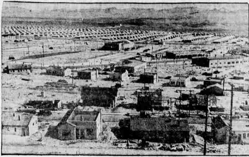
This view shows a section of Boulder City, Colo., a "model" town built about eight miles from the Hoover dam to house workers employed on the project. Thirty-five hundred men and their families live there, the workmen being transported to and from their work in buses.
