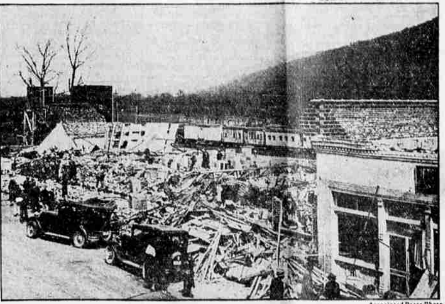
Four persons were killed when a hosiery mill in Paint Rock, Ala., was struck by one of the tornadoes which caused widespread damage and loss of life in the south. The ruins of the mill are shown above.
