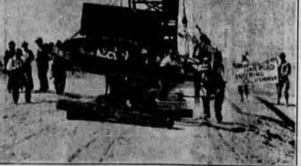
The Great Northern, building a line through southern Oregon and northern California to connect with the Western Pacific, moving its construction equipment across the state line.
