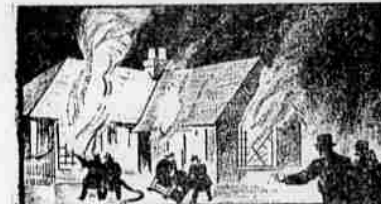
"Then it happened! A faulty chimney was responsible. We stood helplessly while the flames, in a short half hour, badly damaged our home and the belongings it had taken us fifteen years to accumulate."
