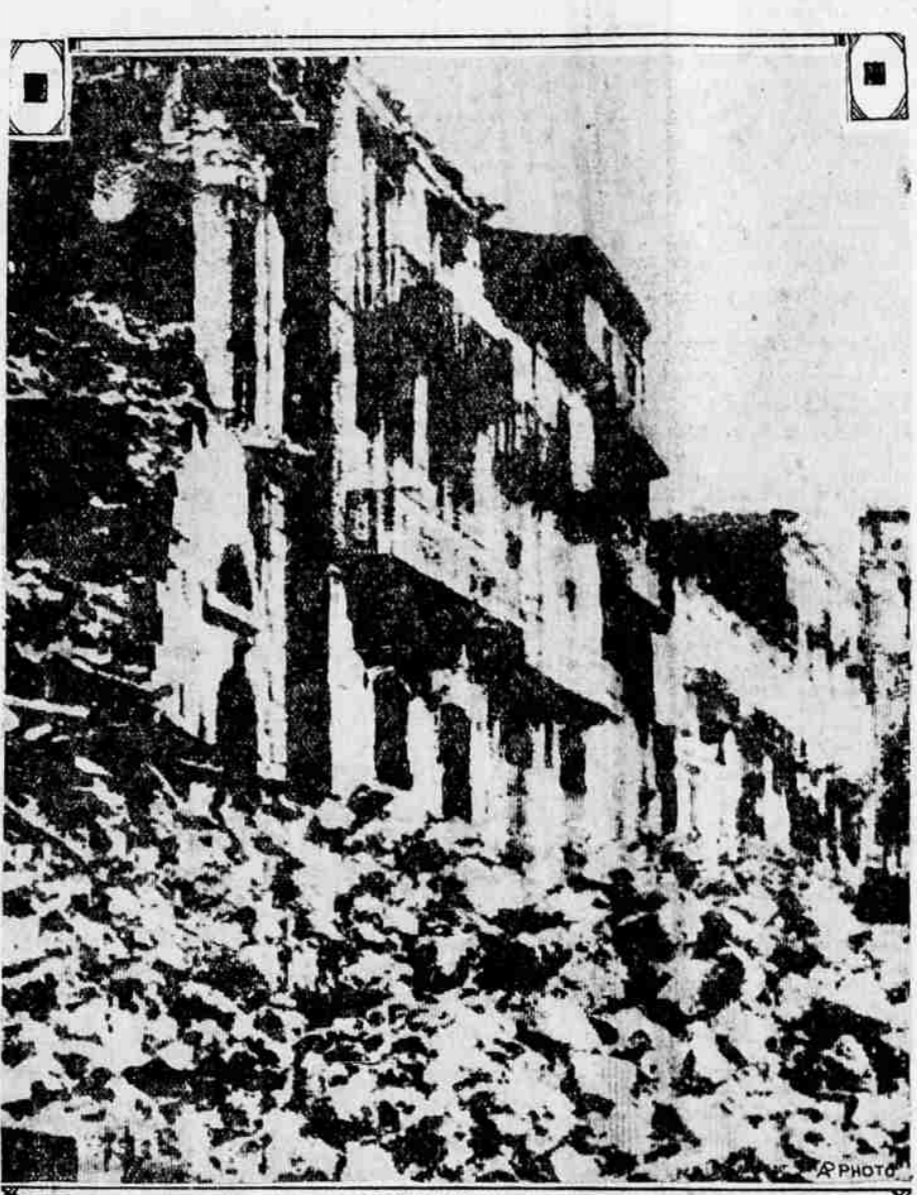
Associated Press photo radioed from London shows ruins caused by earthquake in Maffi, Italy. Maffi was one of the hardest hit towns.
