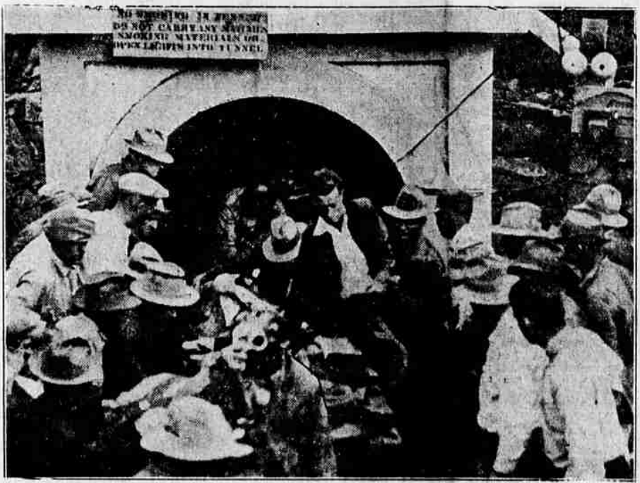
Rescue squads bringing out victims of blast in Mameda county tunnel of San Francisco water department. Seven men lost their lives and one was seriously injured.
