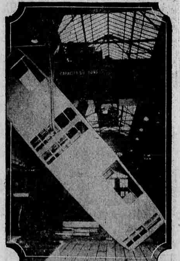
ALLEZ-OOP, HEAVE! Sure to break the grocer's scales is this steel skeleton, weighing something over 50 tons. This frame, shown being lifted into place, is to be part of the stationary element for a big hydro-electric generating unit which will produce 57,000 horsepower of energy at a New York generating station.
