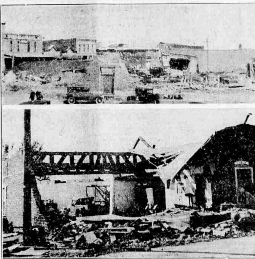
Striking Wagon Mound, N. M., (lower) a tornado caused damage estimated at $150,000 and injured a score. Two men lost their lives in the building shown above.
