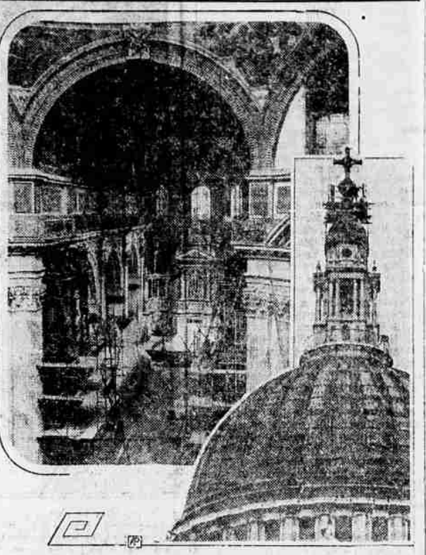
An idea of the extensive repairs and restorations to the interior of St. Paul's cathedral, London, is given at the left. At the right workmen are putting pure gold leaf on the cross atop the lofty dome.
