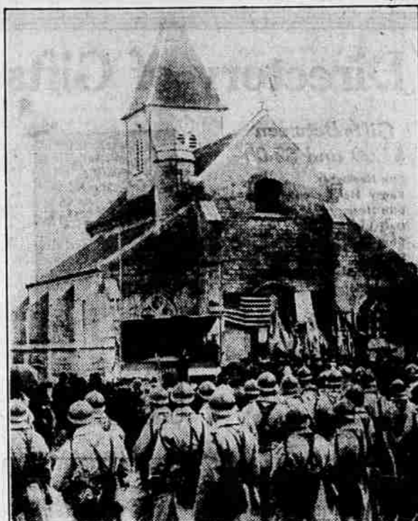
Above is a church presented by the 26th division, United States army, to the town of Belleau, France, where the regiment was encamped for a long time during the late war.
