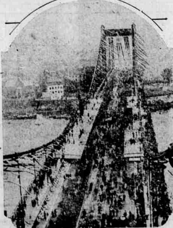
GERMANY'S LARGEST SUSPENSION BRIDGE , one of 32 along the historic Rhine, is shown above, with streamers flying during elaborate dedication ceremonies. It is 4300 feet long and connects Cologne and Muhlheim.
