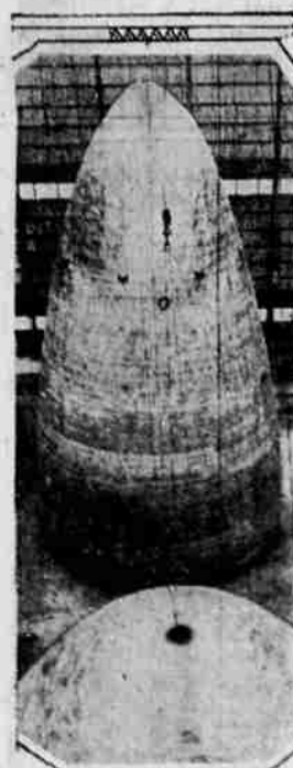
A "TIN AIRSHIP" for the United States Navy was built in sections standing on end in a Detroit factory. One of the sections of the all-metal dirigible is pictured in construction here.
