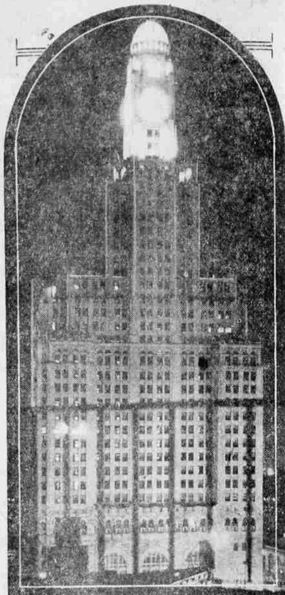
LIGHT BENDS AROUND A CURVE HERE. The 36-foot dome of the new Williamsburgh bank building in Brooklyn is floodlighted internally. Such a procedure by General Electric engineers solved the problem of how to make light "bend" around a curve to light the dome, built not of glass but horizontal metal louvers.
