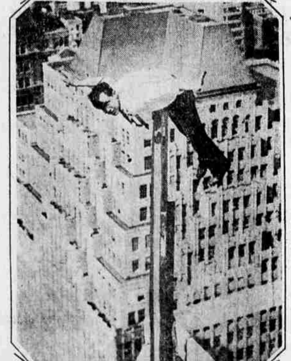
YES, A WAY TO KEEP COOL, but not the best way in the world to most folks. Billy Bomar, circus daredevil, is pictured doing his acrobatic stunts on the scaffolding of a 44-story building under construction in New York. Wolta life!
