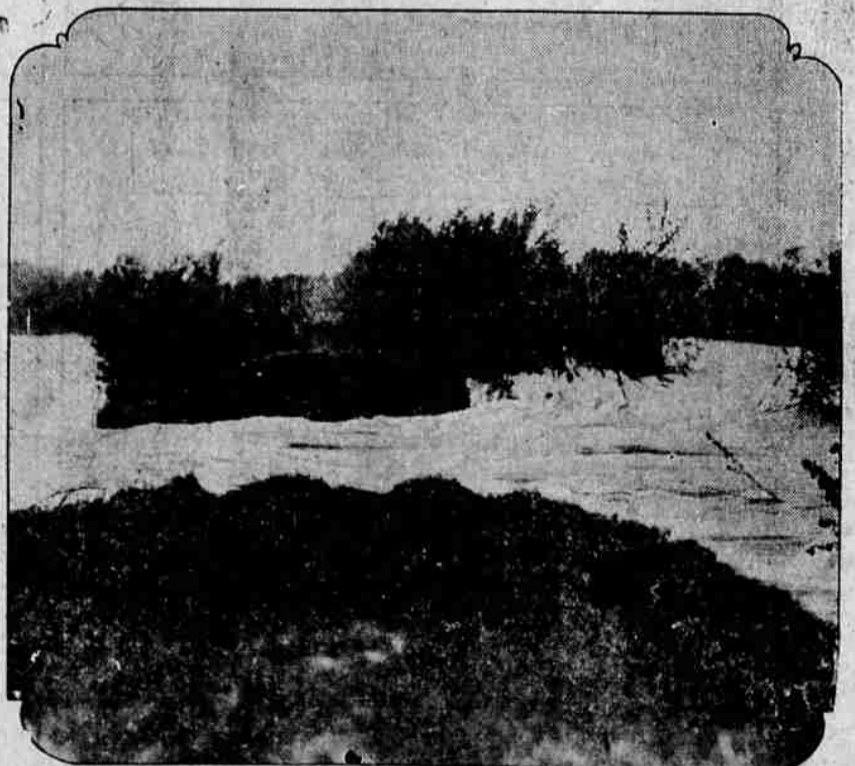
A TINY RIVULET SOON BECOMES A TURBULENT, RUSHING STREAM of water when a levee weakens and thousands of acres are inundated with a waste of millions of dollars. A break in the dike at South Quincy, Illinois, is pictured here.
