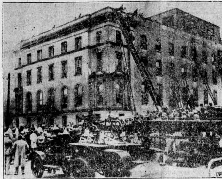
General view of the building after the blast and fire had snuffed out many lives. A large number of patients were rescued from the roof. (Picture by telephoto from Cleveland.)
