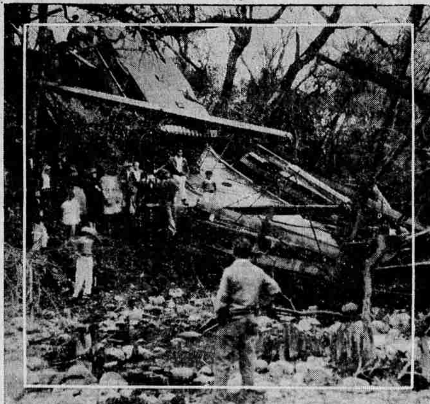
TWO COUNTIES COULDN'T AGREE who should pay for the repair of an old wooden bridge on a county line near Palo Alto, Calif. The result: the bridge, unrepaired, gave way the other day beneath a heavy sight-seeing bus, and 17 occupants narrowly escaped serious injury. Here's what it looked like after the crash.
