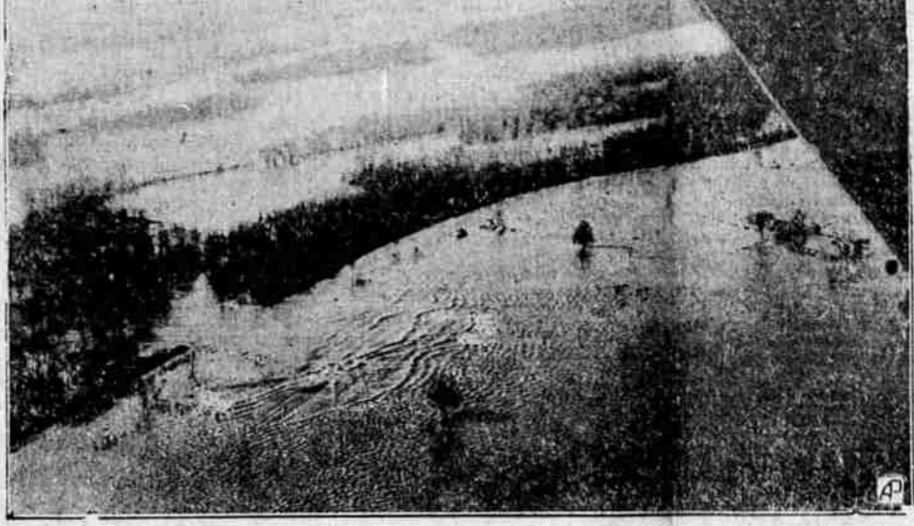
This aerial picture shows the Mississippi river pouring through a break in the levee near the Indian Crave drainage district north of Quincy, La. Thousands of acres have been inundated. The gap in the levee was more than 200 feet wide when this photograph was taken and has been widening rapidly.
