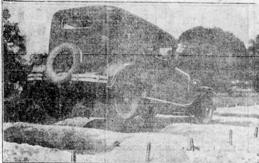
Oldsmobile Six being tested on "worst road in the world" at General Motors Proving Ground for riding qualities, spring action and efficiency of its hydraulic shock absorbers.
