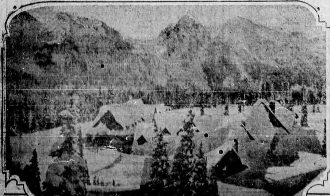
WRAPPED IN A DEEP SNOW BLANKET, WITH BROODING MOUNTAIN PEAKS in the background, Para's Valley Inn, in Rainier National Park, presents a strange picture in mid-winter. Plans are now being made for installing an aerial cable to carry tourists to the inn when, as now, it is covered with 20 feet of snow.
