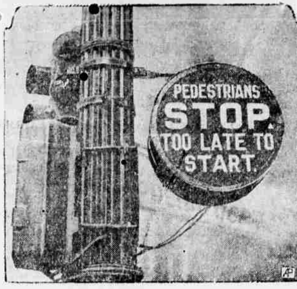
Detroit is trying out a new traffic control signal, designed to safeguard pedestrians crossing busy thoroughfares. It warns those about when it is too late to beat cross traffic.
