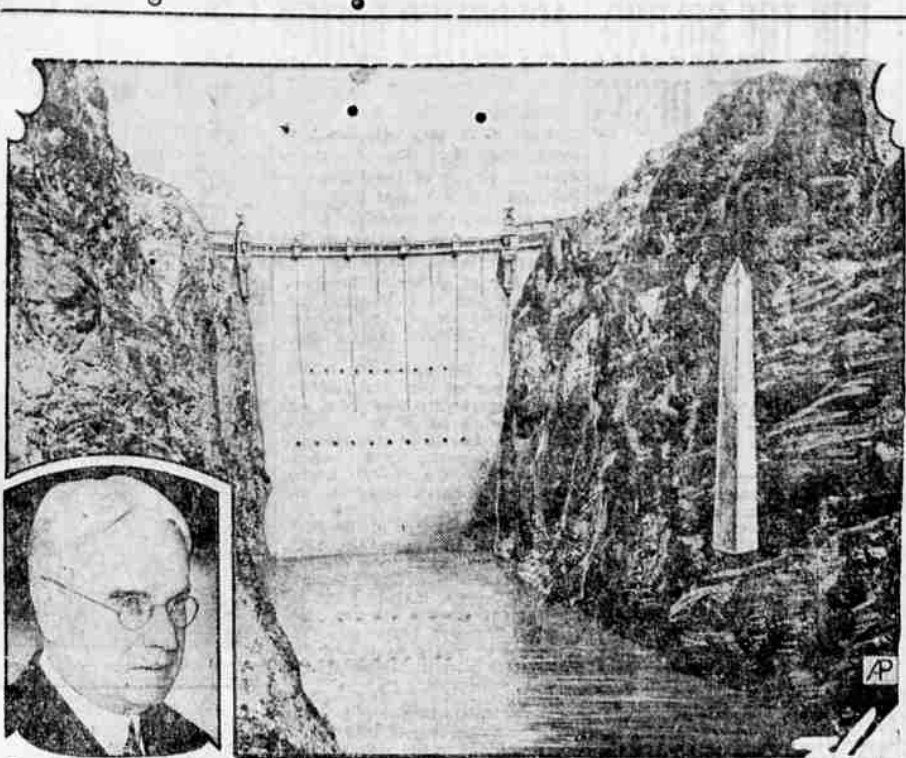
Boulder Dam, the construction of which has been authorized by congress, would put a halter on the tumbling and destructive Colorado river. The dam will be a concrete wall, 560 feet high, located at Black Canyon (as in sketch above). It would impound 26,000,000 acre feet of water and store 20,000,000 acre feet. Senator Hiram Johnson (inset) of California has been chief champion of the legislation.
