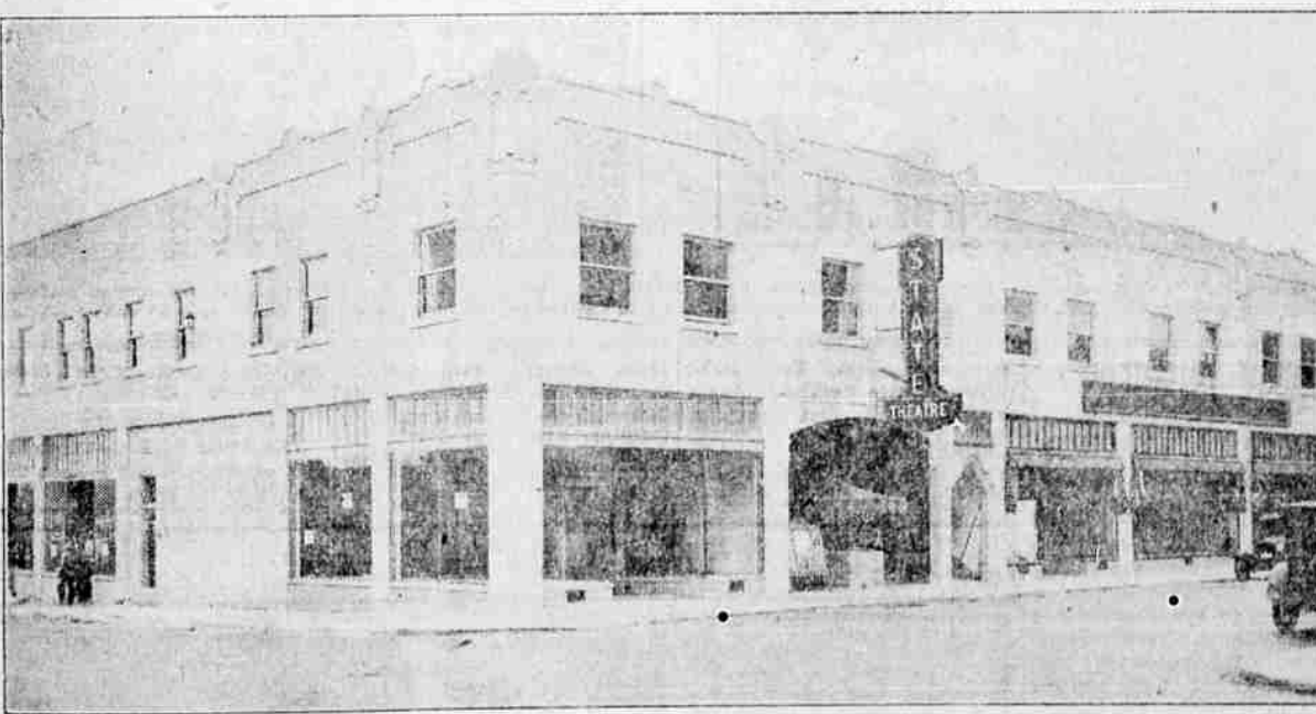
One of Medford's newest and most imposing business structures is the Leverette building which was completed during 1928 at the corner of Eighth Street and Central Avenue. The building was erected by Walter Leverette, Medford realtor, and houses the Montgomery Ward & Company, the State theatre, Bursell's Women's Ready-to-Wear store, E. C. Corn's real estate office, and the Wardwell Fur company.
