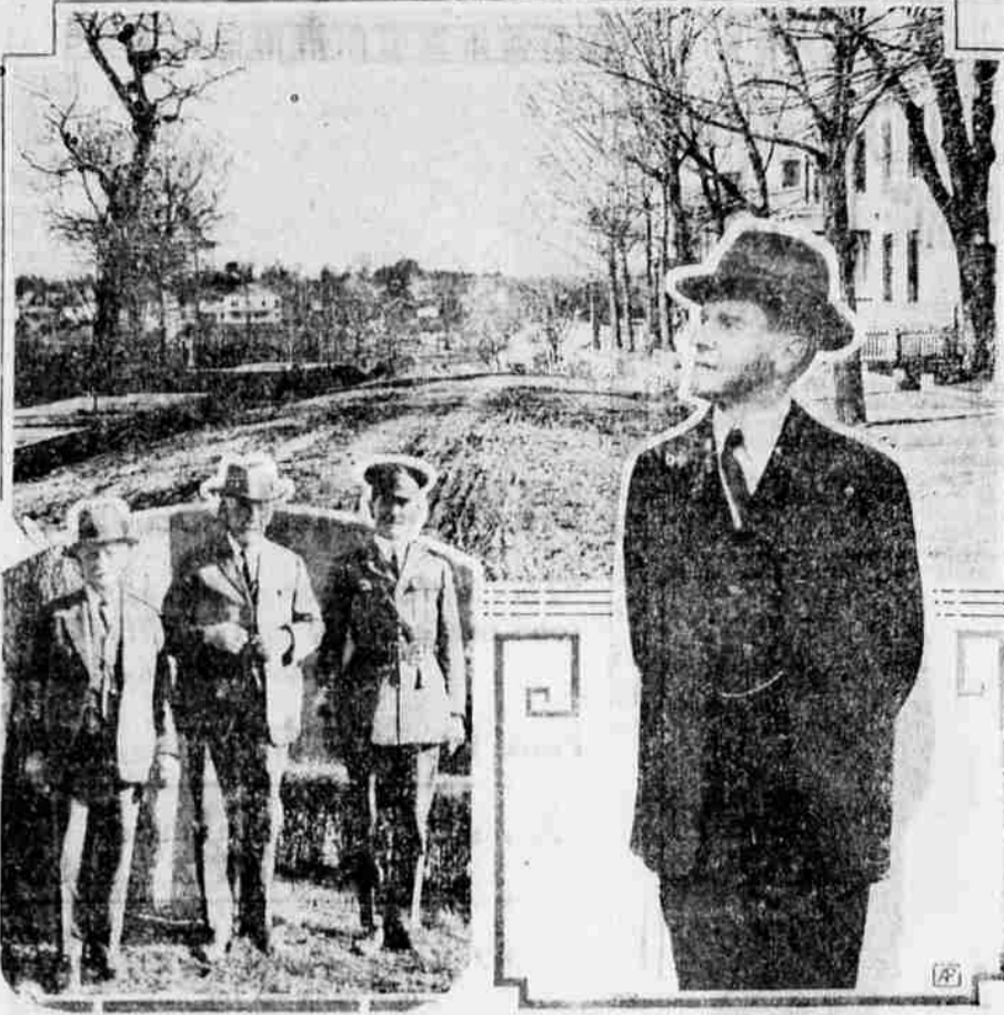
Construction work on one of the greatest battle memorials in the country was formally launched by President Coolidge at Fredericksburg, Va. The project will embrace five Civil war battlefields in a system of parks and roads. Hanover street (above) over which seven divisions of Union troops attacked ineffectively to take Marye's Heights is little changed. On the park commission is Gen. John L. Chen, "the drummer boy of Shiloh." He is to the left of the group below. Others, left to right, are V. M. Fleming, Confederate veteran, and Capt. George F. Hobson, in charge of construction.
