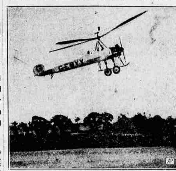
This autogyro flying machine piloted by J. De La Cierva, its inventor, averaged 100 miles an hour on a test flight from Croydon field, England, to LeBourget, Paris. The machine which carries four huge blades rotating on its top is capable of making a practically vertical landing, eliminating necessity of a large landing field.
