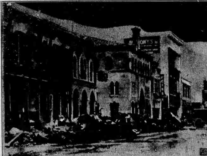
Business center of West Palm Beach, Florida, as left by the West Indian hurricane. Photo transmitted to Pacific Coast by telephoto.
